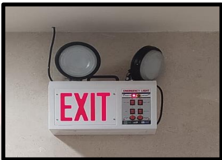
Battery Operated Emergency lights in Corridors/stairs
