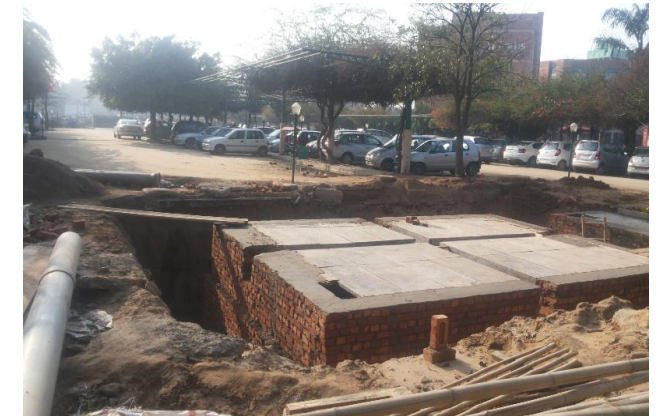
Rain Water Harvesting Pits
