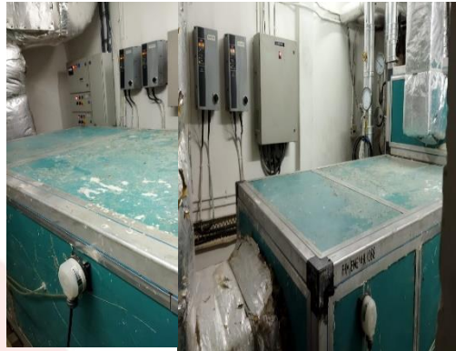
VFD Operated AHU's
