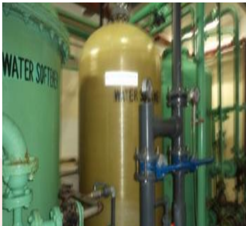
550KLD Sewage treatment plant
