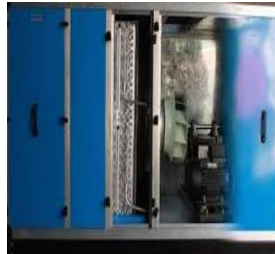
Ahu with EC fans
