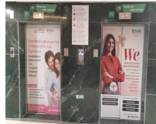
Synchronized Elevators Operations
