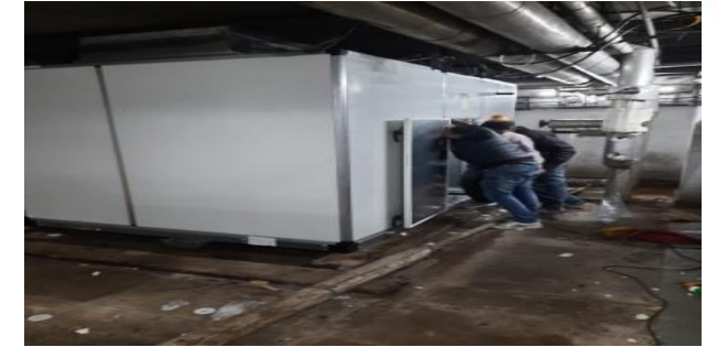
Vintage old inefficient AHU's replacement
