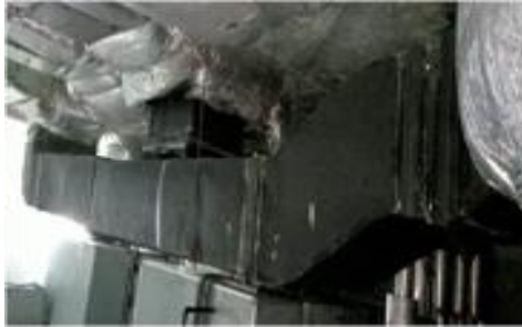
Split AC's replaced with FCU's
